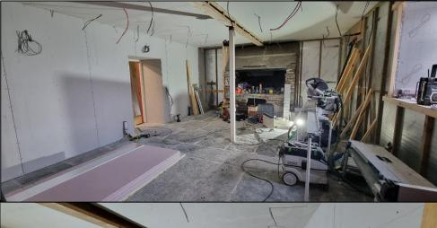
In the restaurant all the walls have been insulated, strapped and lined and plasterboard is being installed, ready for taping and filling.
